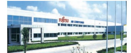
Fujitsu General (Shanghai) Co., Ltd. (China)
