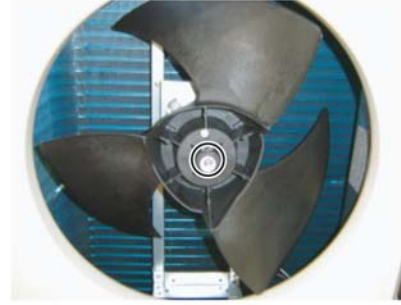
Remove the Hex Socket Screw. And remove the PROPELLER FAN. Note at the installation. Insert propeller Fan and Motor shaft reference D cutting position. And the tightening torque at the installation. Tightening torque is from 10 to 15 N.M.
