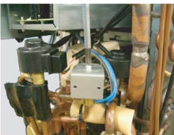
Remove the mounting screw.
