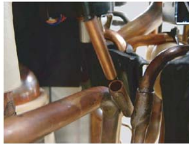
Remove the THERMISTOR SPRING. Remove the THERMISTOR.
