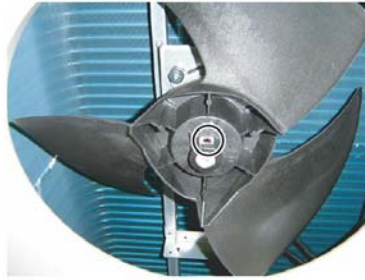
Remove the Hex Socket Screw and remove the PROPELLER FAN. Note at the installation. Insert propeller Fan and Moter shaft reference D cutting position. And the tightening torque at the installation. Tightening torque is from 10 to 15Nm.
