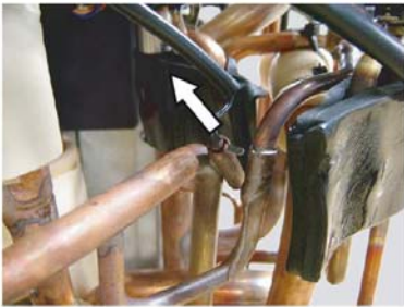
Remove the THERMISTOR SPRING. Remove the THERMISTOR.
