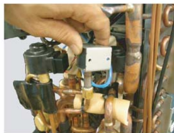
Remove the SOLENOID COIL.
