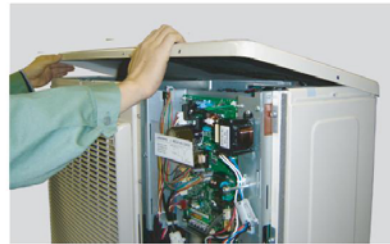
Remove the TOP PANEL.
