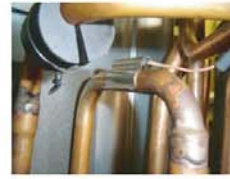
Remove the Thermistor (Discharge).
