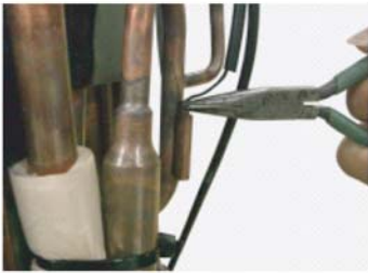
Remove the THERMISTOR SPRING.
