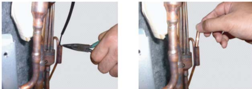
Remove the THERMISTOR SPRING. Remove the THERMISTOR.
