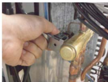
Remove the SOLENOID COIL.
