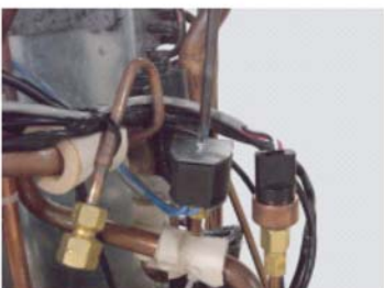
Remove the mounting screw.
