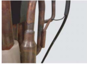
Remove the THERMISTOR.
