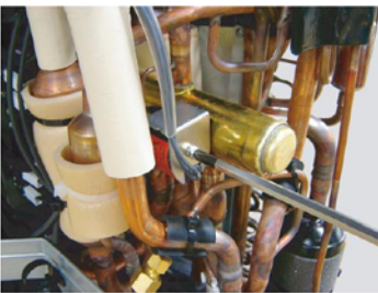
Remove the mounting screw.
