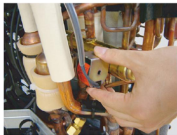
Remove the SOLENOID COIL.
