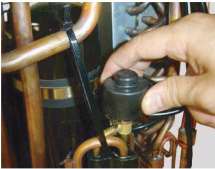
Remove the EEV coil by hand.
