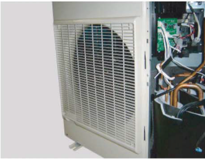
Remove the 4 mounting screws.
