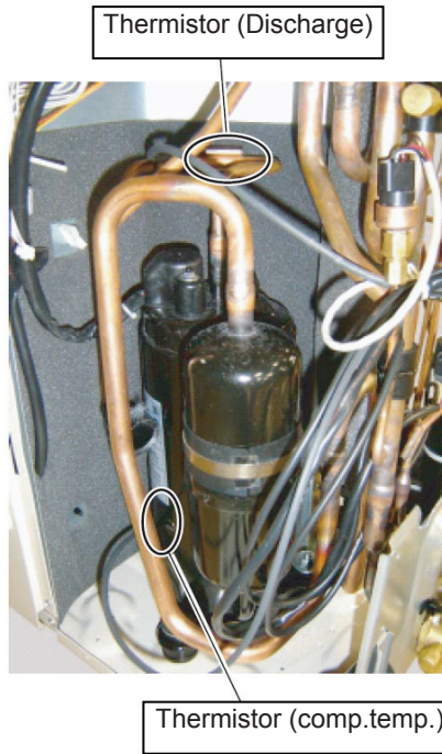
Remove the Thermistor (comp. temp.) and Thermistor (Discharge)
