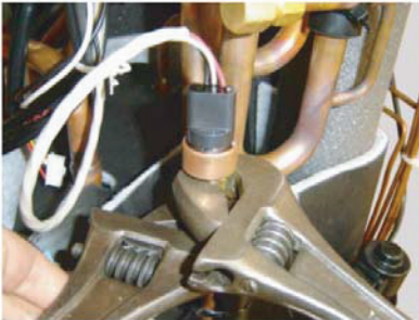
Remove the PRESSURE SENSOR with wrench.
