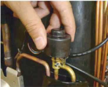
Remove the EEV coil by hand.
