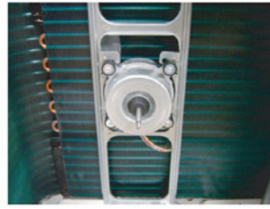
Remove the PROPELLER FAN.
