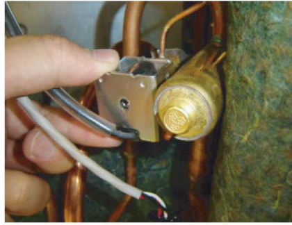
Remove the SOLENOID COIL
