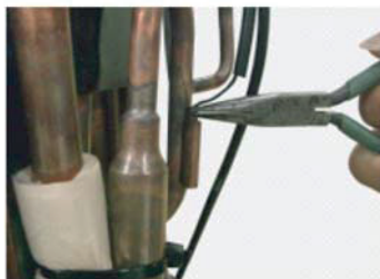
Remove the THERMISTOR SPRING.
