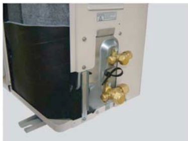
Remove the VALVE COVER.
