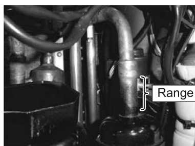
Cut the Suction pipe in this range. Remove the COMPRESSOR.
