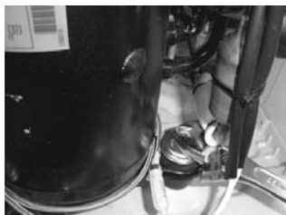
Remove the COMP BOLTS. (3 places)
