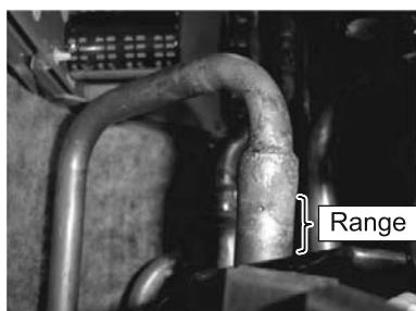
Cut the Discharge pipe in this range.
